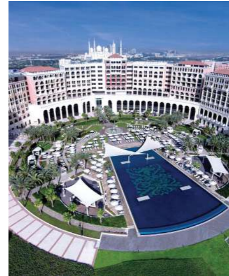
THE RITZ - CARLTON ABU DHABI - GRAND CANAL Abu Dhabi Hotel
